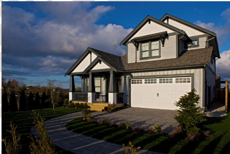
Photo of new leasehold residential unit
